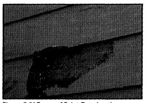
Figure 5.2f Forms of Paint Deterioration: Cracking, Peeling, and Blistering. Courtesy: National Decorating Products Association
