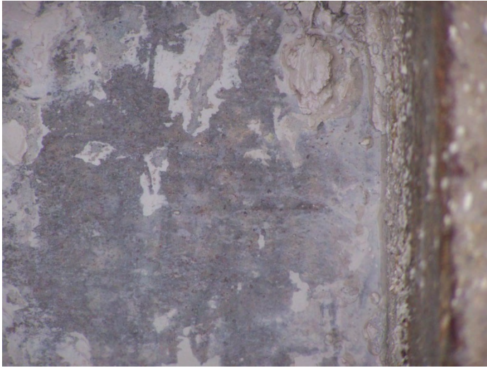
Photograph #13- SWMU #11- South Spray Line Trench Bottom
