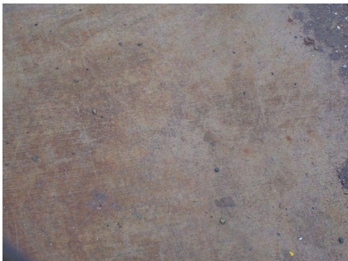
Photograph #11- SWMU #11- South Spray Line Sump Floor
