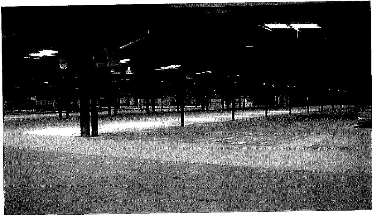
Photo Number: 22 Direction: Facing southwest Description: View of the inside of the main process building
