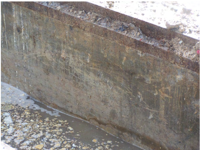
Photograph #8- SWMU #11- Spray Line Sump Walls
