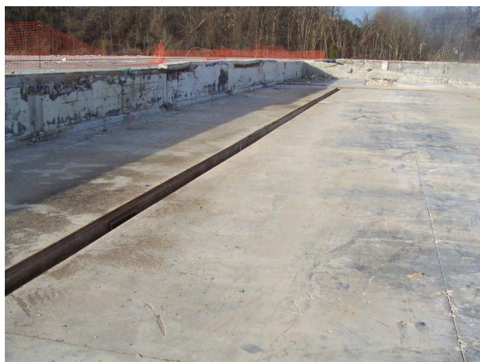
Photograph #5- SWMU #11- Spray Line South Trench Area
