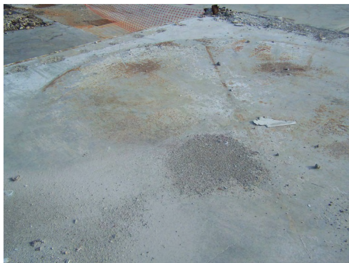
Photograph #3- SWMU #1- WWT System Floor Secondary Containment Area and Wipe Sample #3
