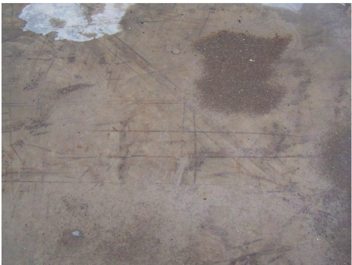
Photograph #10- SWMU #11- North Spray Line Sump Floor
