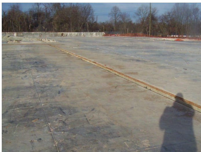
Photograph #6- SWMU #11- Spray Line North Trench Area
