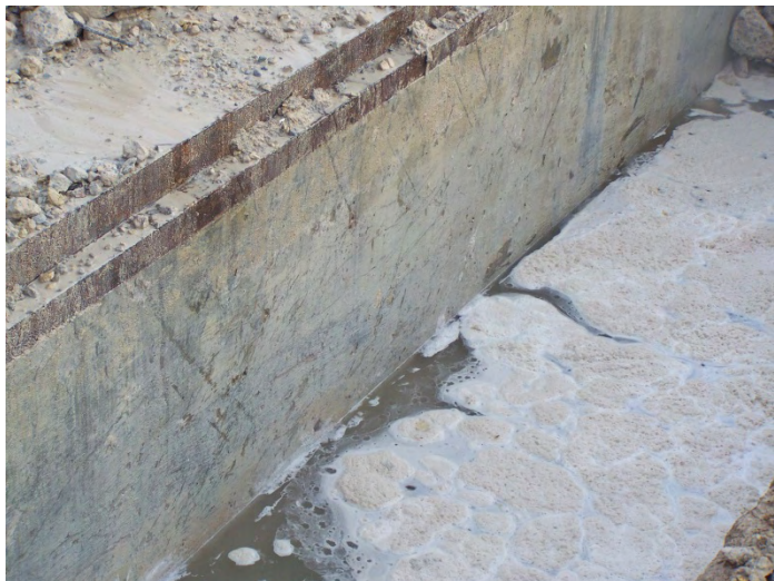
Photograph #7- SWMU #11- Spray Line Sump Walls
