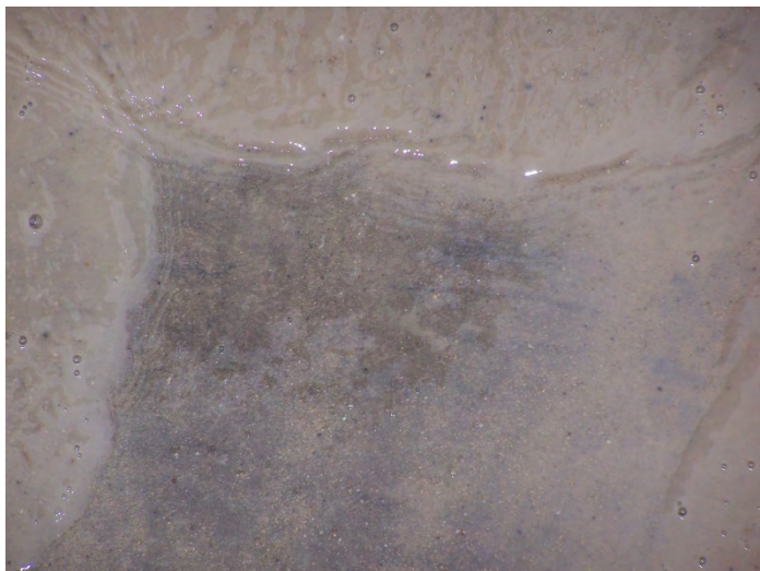
Photograph #9- SWMU #11- North Spray Line Sump Floor
