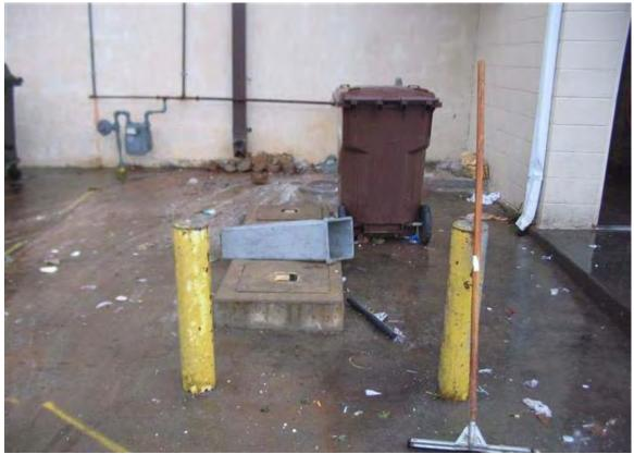
Photograph #11- Food grease trap and grease bin at rear of Building 1 for restaurant tenant space
