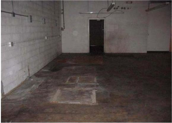
Photograph #15- Corroded concrete in area of former machinery inside the former dry-cleaner tenant space
