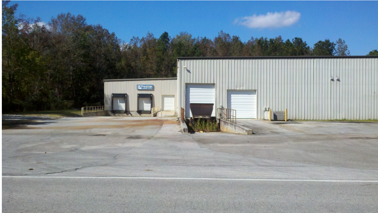
Photograph 8: Loading docks along the east side of the manufacturing area as viewed from the east.
