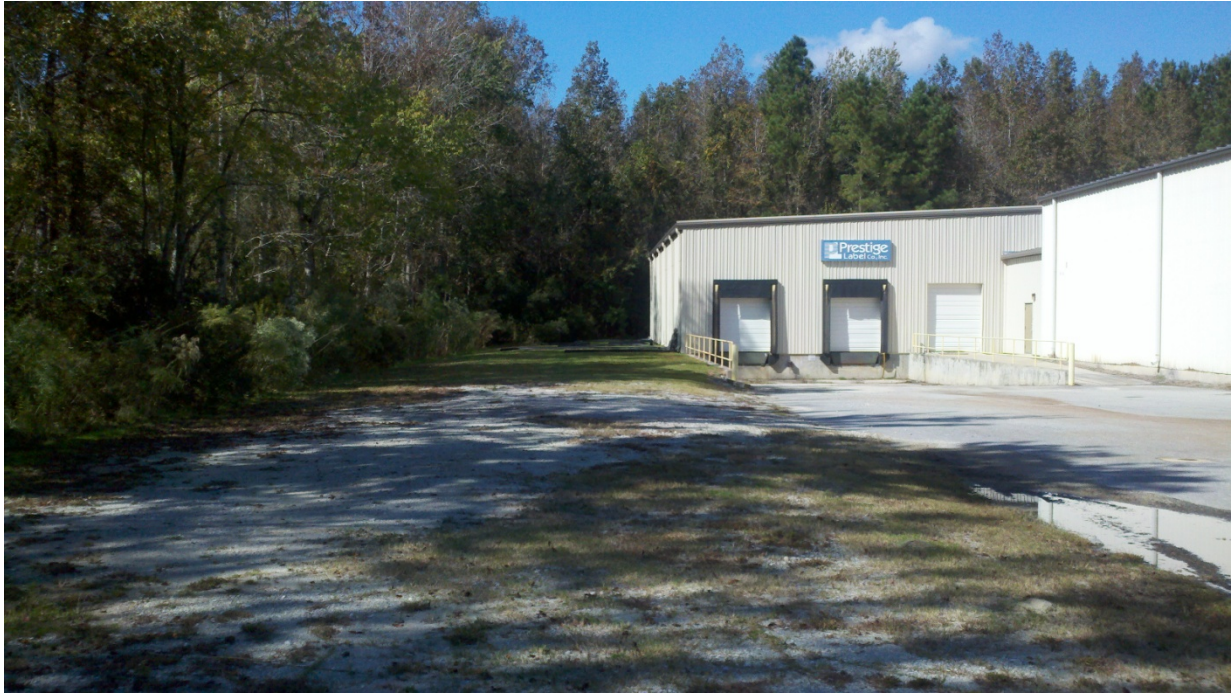
Photograph 1: South side of the site as viewed from the east.
