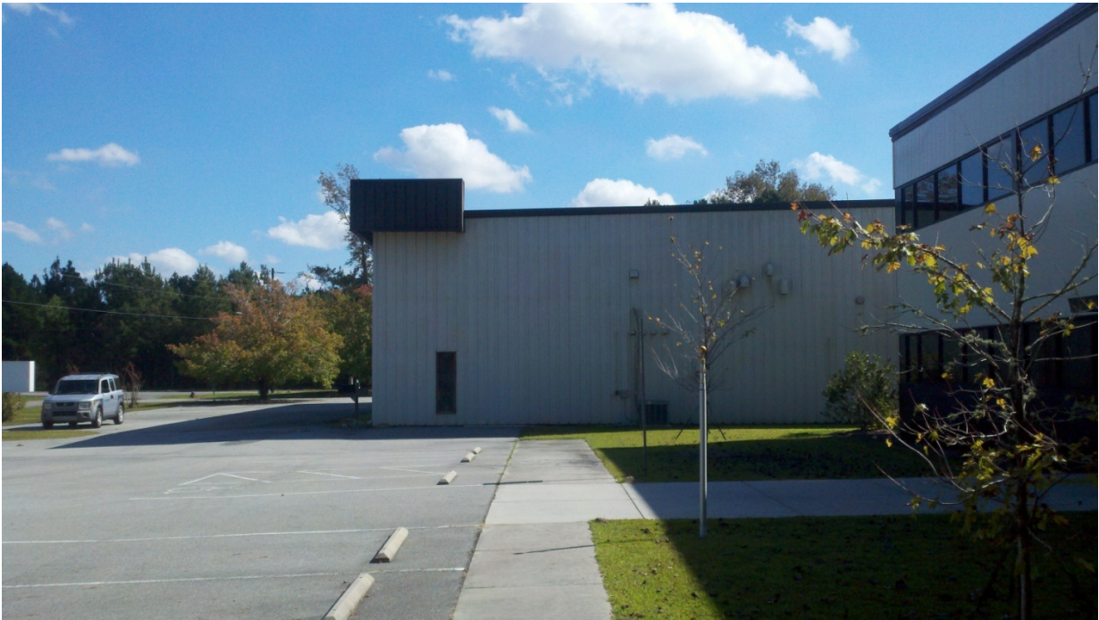
Photograph 14: West side of the office area as viewed from the west.
