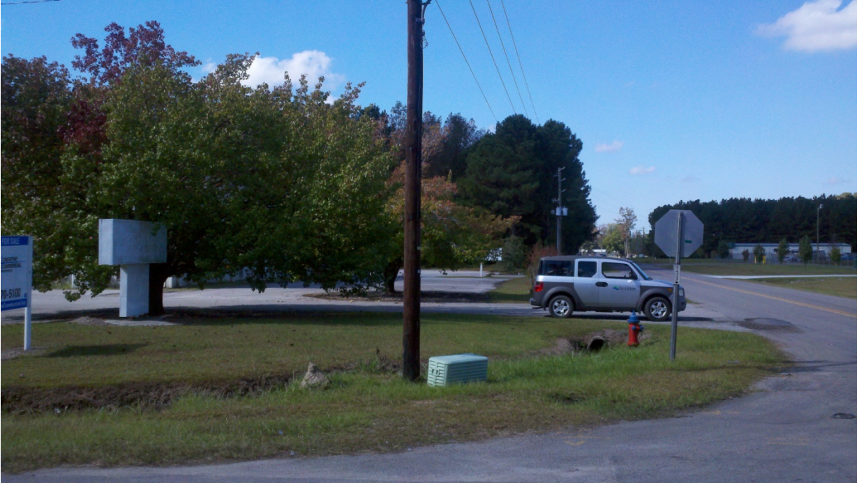
Photograph 11: North side of the site as viewed from the east.
