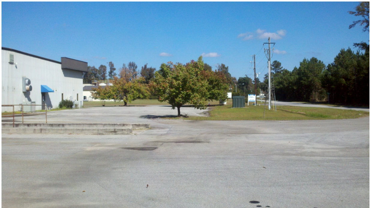
Photograph 6: East side of the manufacturing and office area building as viewed from the south.
