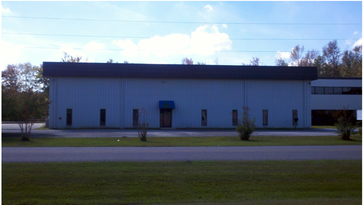
Photograph 10: North side of the office area as viewed from the north.
