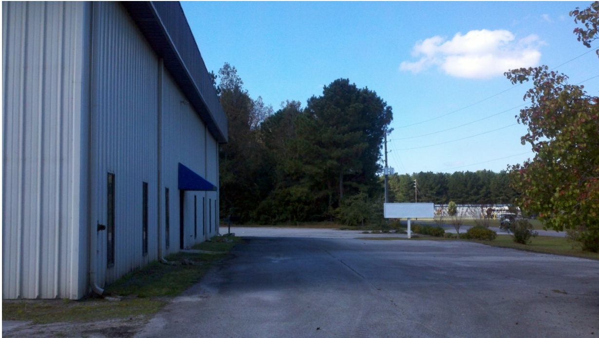
Photograph 9: North side of the office area as viewed from the east.
