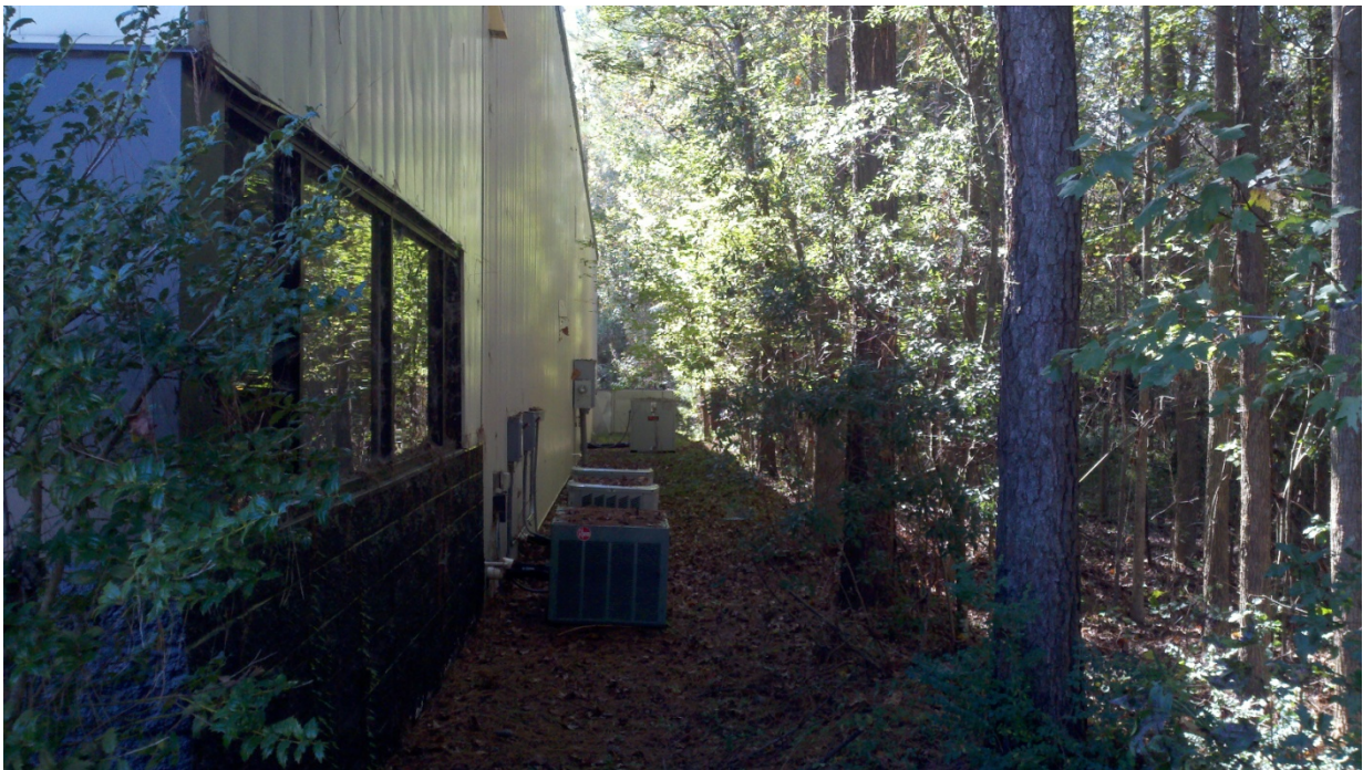
Photograph 16: West side of the new building as viewed from the north.
