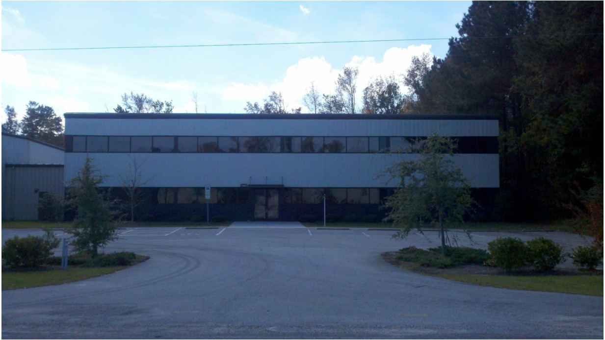
Photograph 13: North side of the new building as viewed from the north.
