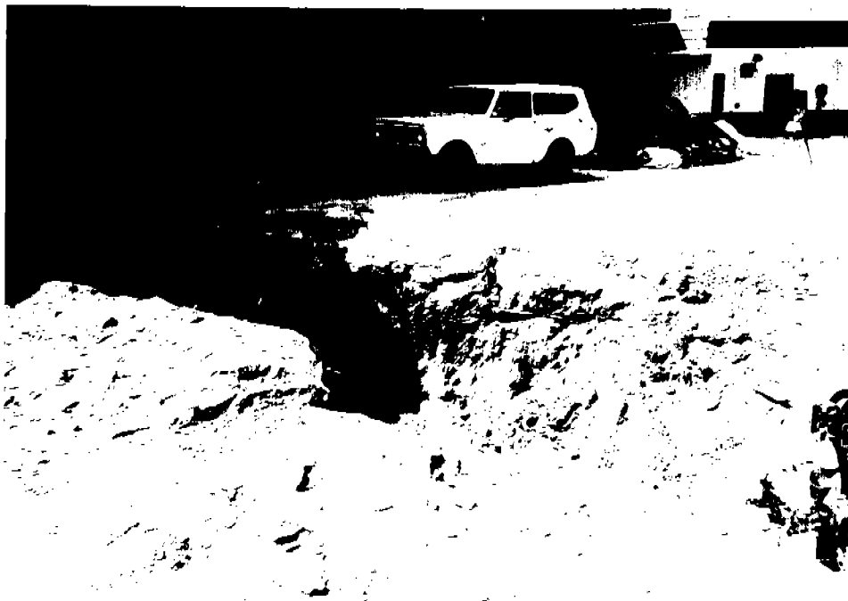
UST excavation area
