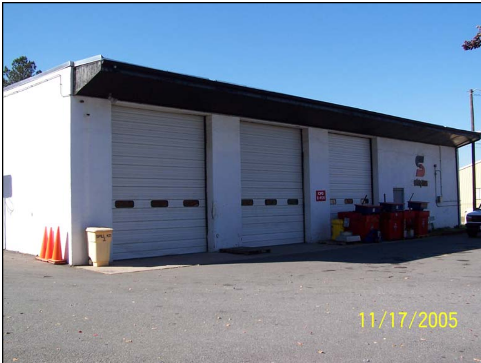
Photo # 4: Class 1B Flammable Container Storage Warehouse looking south (RCRA permitted Class 1B Container Storage Area located inside)
