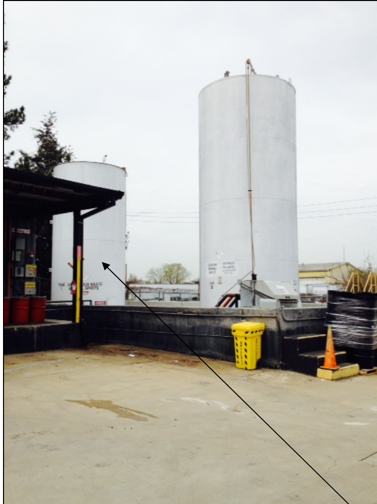
Photo # 12: Parts Washer Solvent Tank Farm looking west. RCRA permitted Used Parts Washer Storage Tank (S02) located on left inside tank farm. Photo taken 4/10/14.
