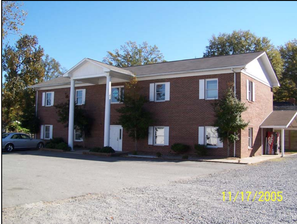
Photo # 3: View of Office Building looking east.
