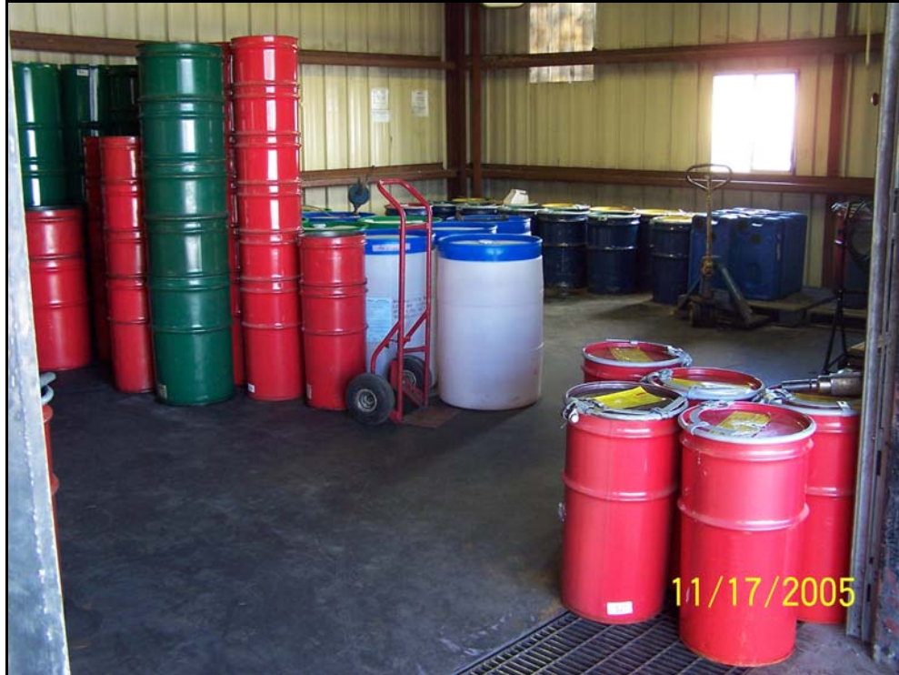
Photo # 11: Interior view of Non-Ignitable Container Storage Warehouse looking west (RCRA permitted - S01)
