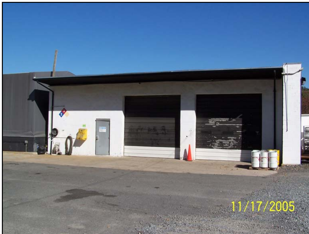
Photo # 6: Exterior view looking northeast at Class 1B Container Storage Warehouse. RCRA permitted Class 1B Container Storage Area (S01) located inside.
