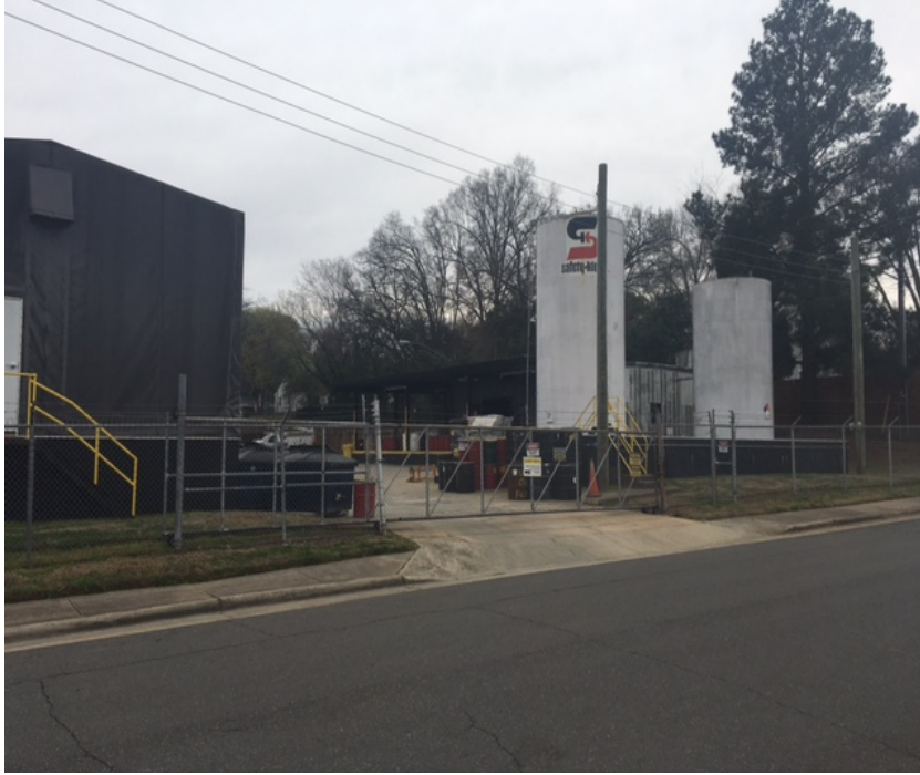
Photo # 14: View looking south of secondary Facility access gates (truck gate and man gate) located off Yadkin Avenue. Photo taken 2/27/17.
