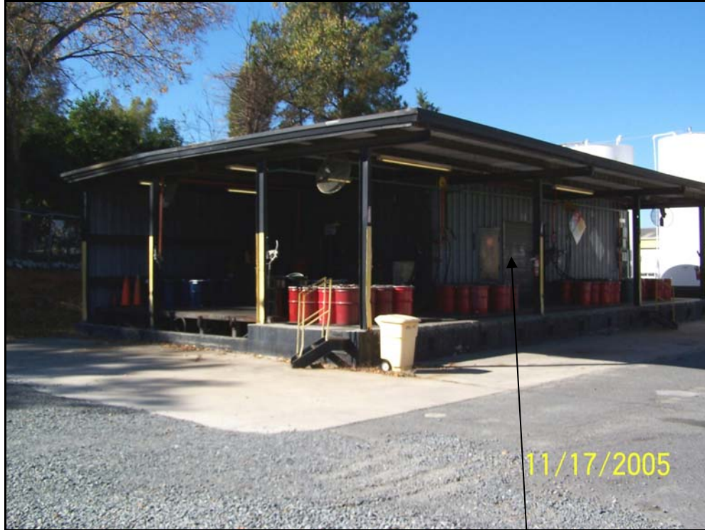
Photo # 9: Non-Ignitable Container Storage Warehouse (S01) / Return and Fill Area looking west.
