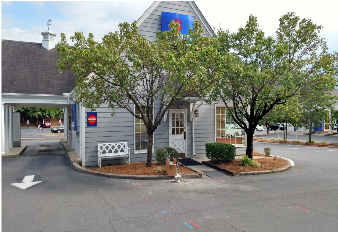
Photograph 3: VMP-1, during sampling activities.
