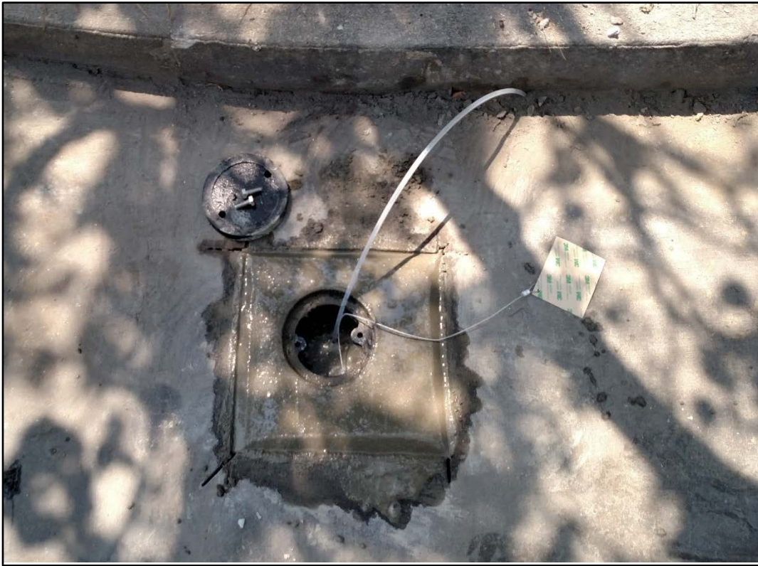
Photograph 1: VMP-1, following installation.
