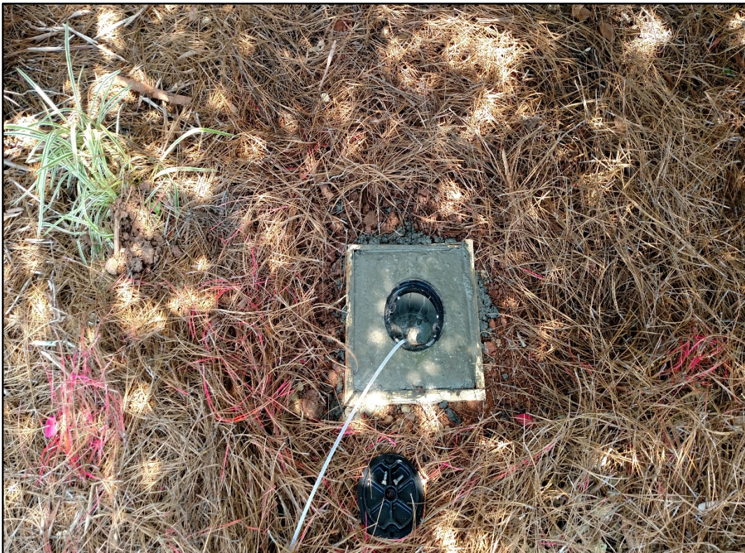
Photograph 2: VMP-2, following installation.
