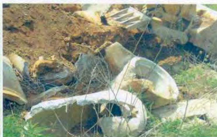
Photo D: Concrete culvert on ground surface at TP-11.
