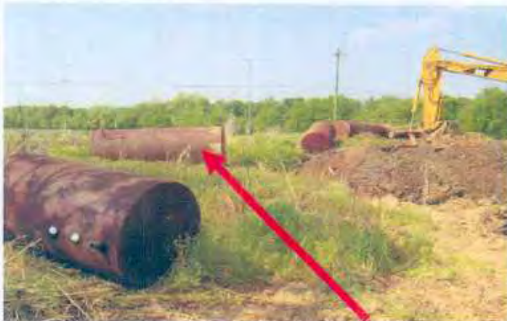
Photo O: Tank containing approximately 11 inches of gas and water..
