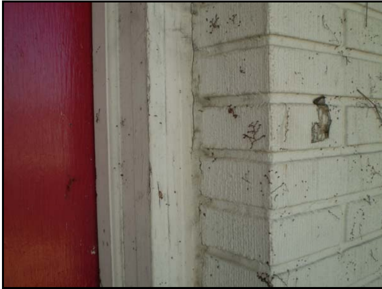
Photograph 5: View of door caulk.
