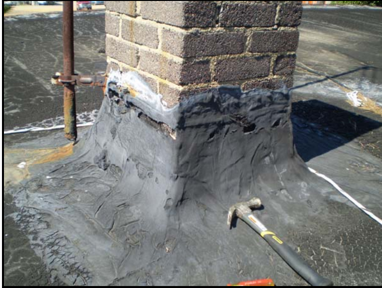
Photograph 3: View of chimney caulk.
