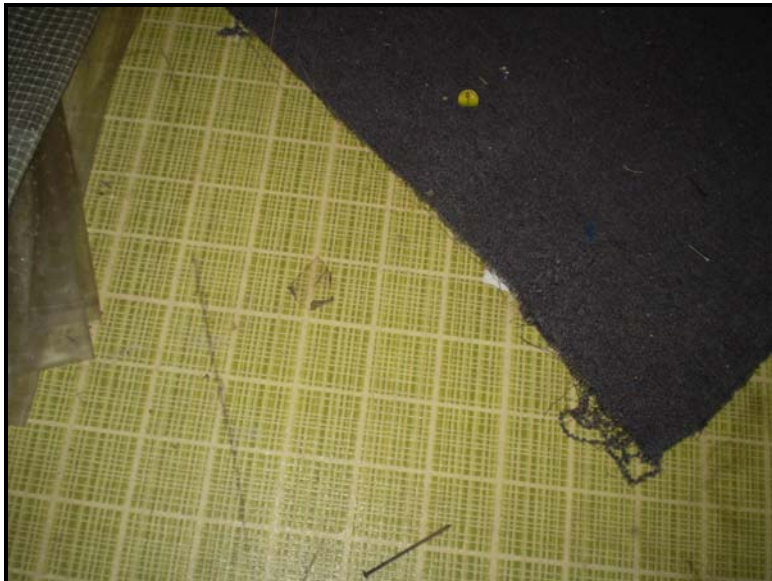
Photograph 4: View of pantry linoleum.
