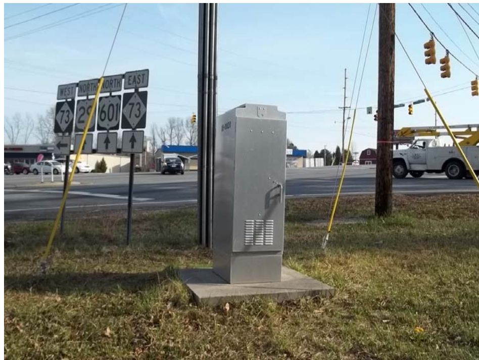
Photograph 10: Utilities at corner of Concord Parkway North and Florence Avenue.
