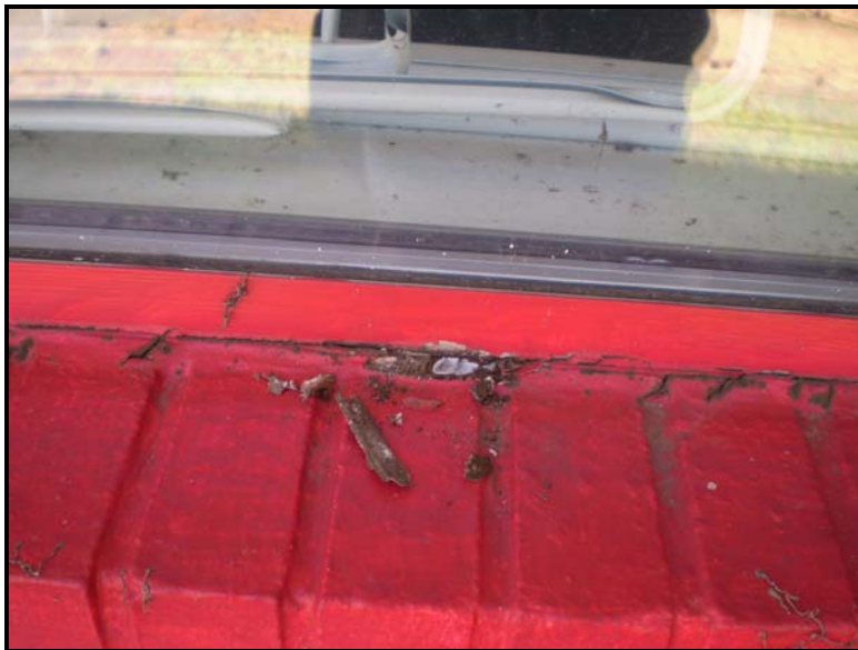
Photograph 6: View of window caulk.
