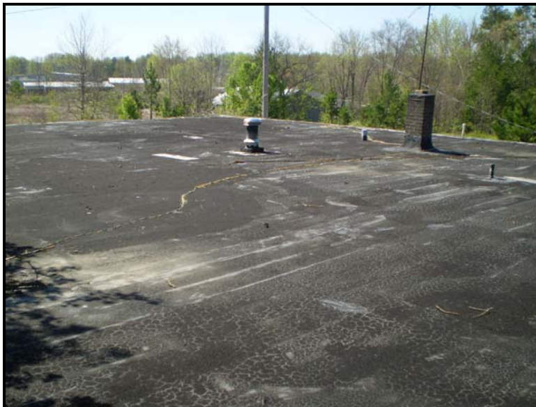
Photograph 2: View of roof.
