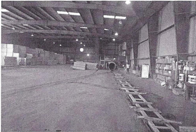
Drip pad building and charge cart
