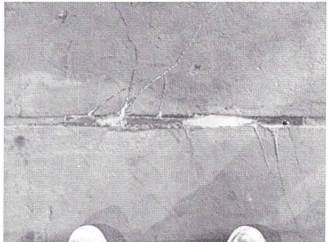
Resealed (repaired) expansion joint
