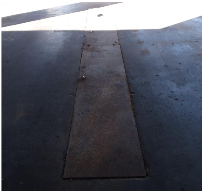
Photo 8 – Sump located on the floor of the northeast building.
