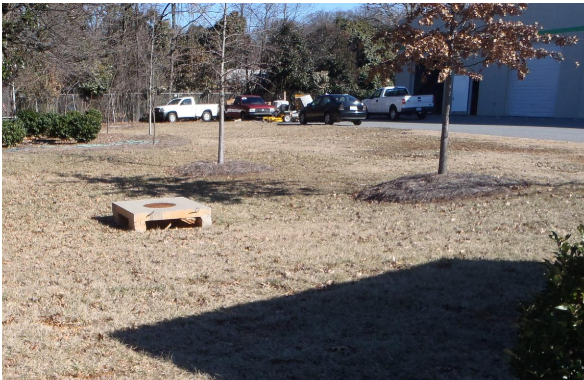
Photo 10 – Storm drain located in the north-central part of the subject site.
