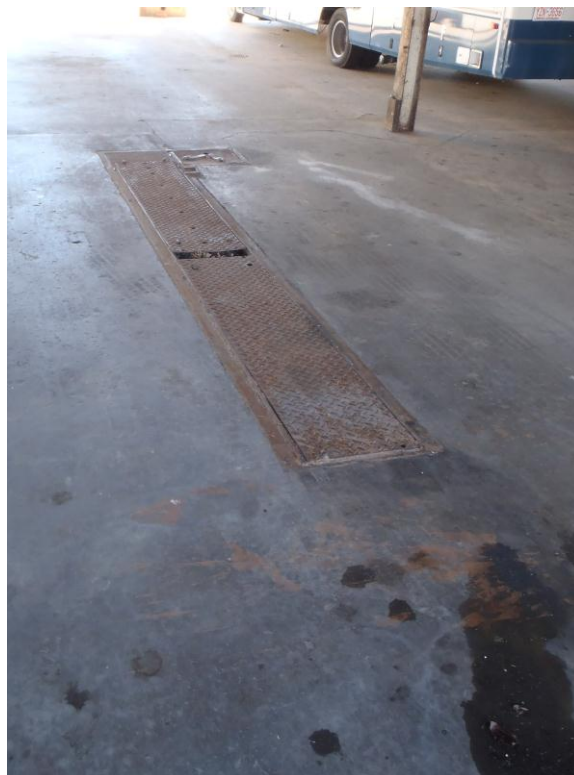
Photo 6 – Possible automobile lift and staining inside the northeast building.
