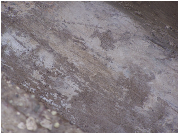
Photograph #12- SWMU #11- North Spray Line Trench Bottom
