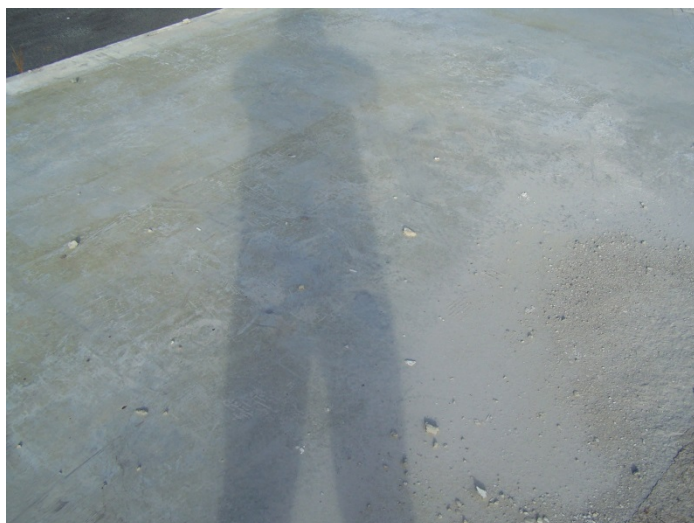
Photograph #4- SWMU #1- WWT System Floor Area and Wipe Sample #4
