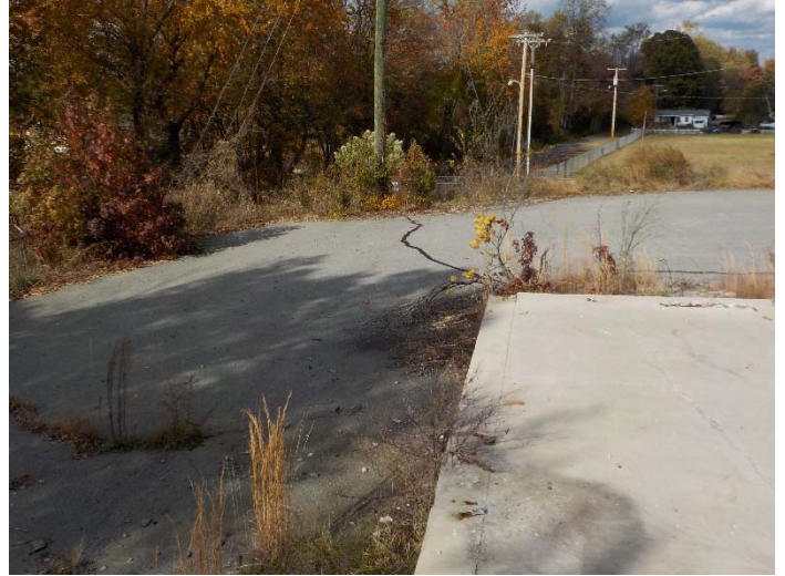
SWMU-9 Area Viewing North
