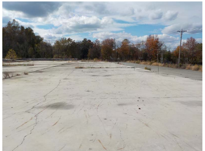
SWMU-11 Area Viewing West
