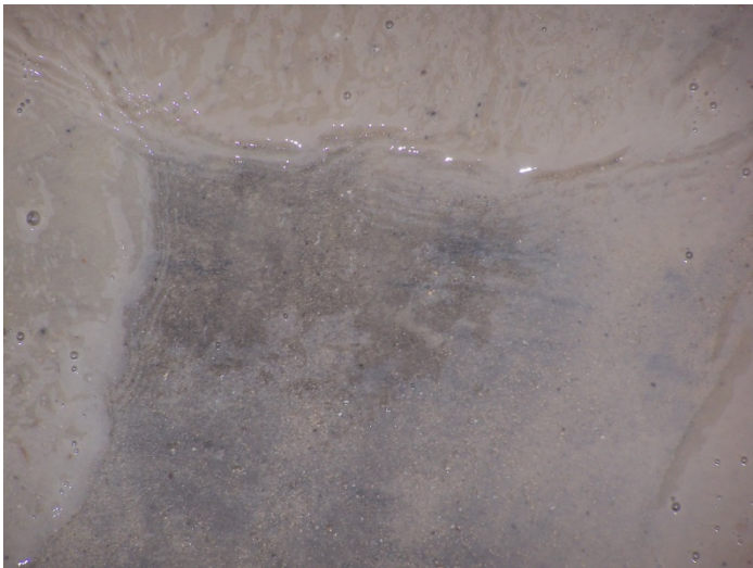
Photograph #9- SWMU #11- North Spray Line Sump Floor
