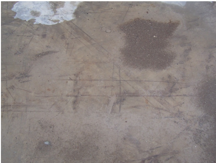
Photograph #10- SWMU #11- North Spray Line Sump Floor
