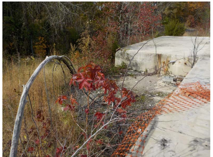
SWMU-4 Area Viewing Northwest
