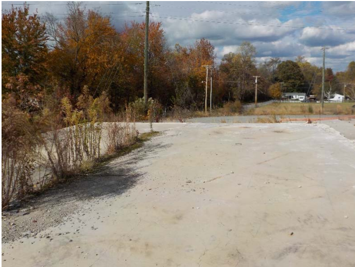
SWMU-1 Area Viewing North
