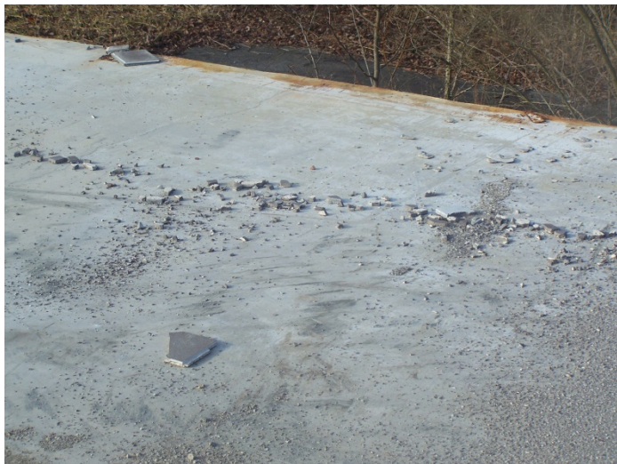
Photograph #1- SWMU #1- WWT System Floor Area and Wipe Sample #1
