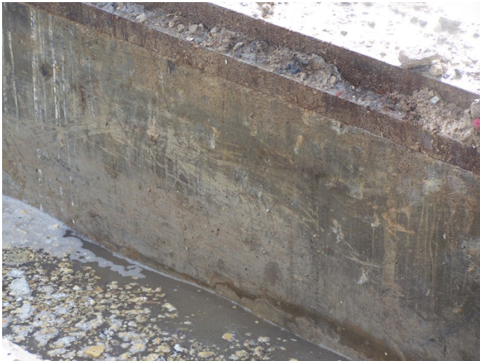
Photograph #8- SWMU #11- Spray Line Sump Walls
