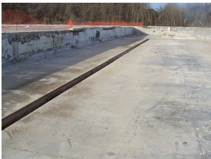
Photograph #5- SWMU #11- Spray Line South Trench Area
