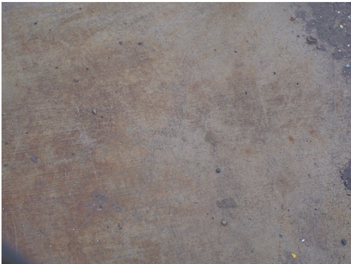
Photograph #11- SWMU #11- South Spray Line Sump Floor
