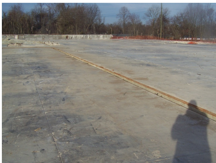
Photograph #6- SWMU #11- Spray Line North Trench Area
