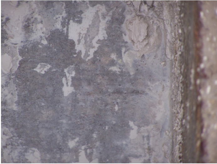
Photograph #13- SWMU #11- South Spray Line Trench Bottom
