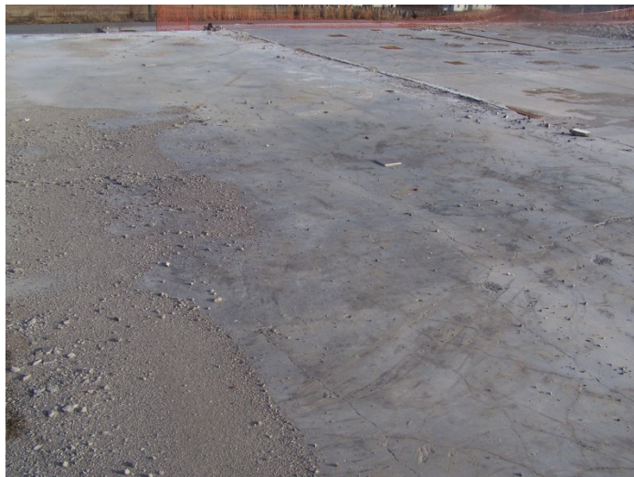
Photograph #2- SWMU #1- WWT System Floor Area and Wipe Sample #2
