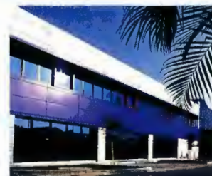
This DuPont Lycra® spandex facility in Singapore is part of a major expansion of manufacturing capacity in the fast-growing Asia/Pacific region.
