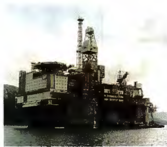
The giant Heidrun oil field in the Norwegian sector of the North Sea is being developed using a tension leg platform, technology developed by Conoco to bring within reach petroleum deposits beneath the seabed in very deep waters.
