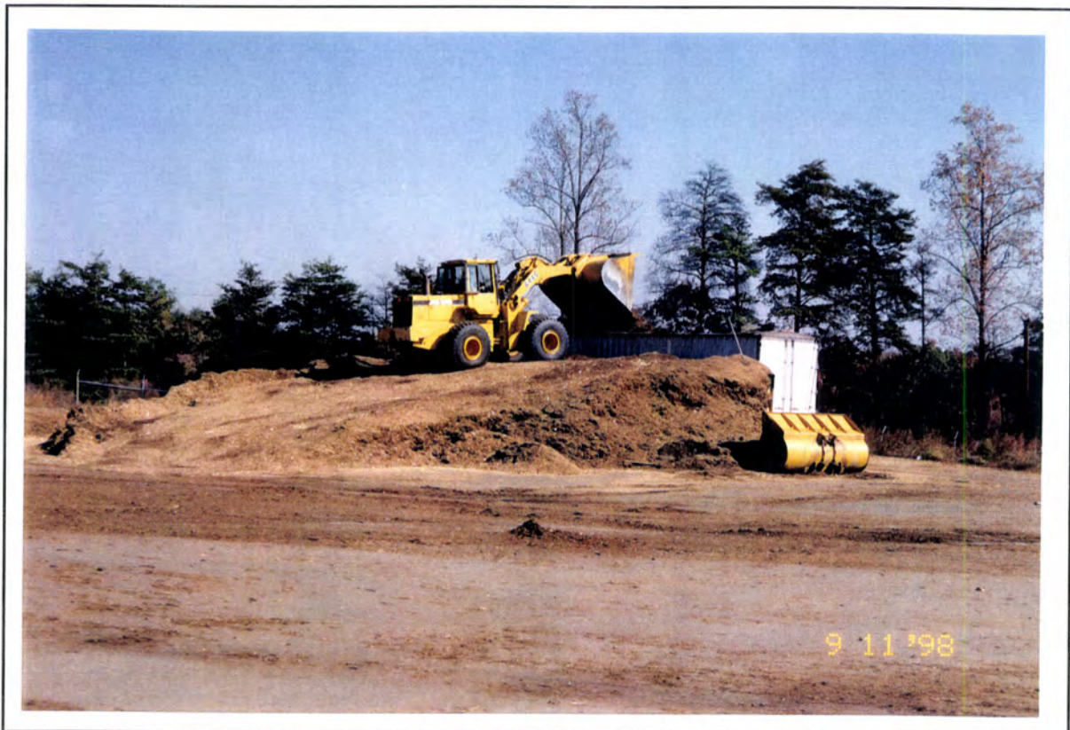
Loadout Area, looking northeast.
