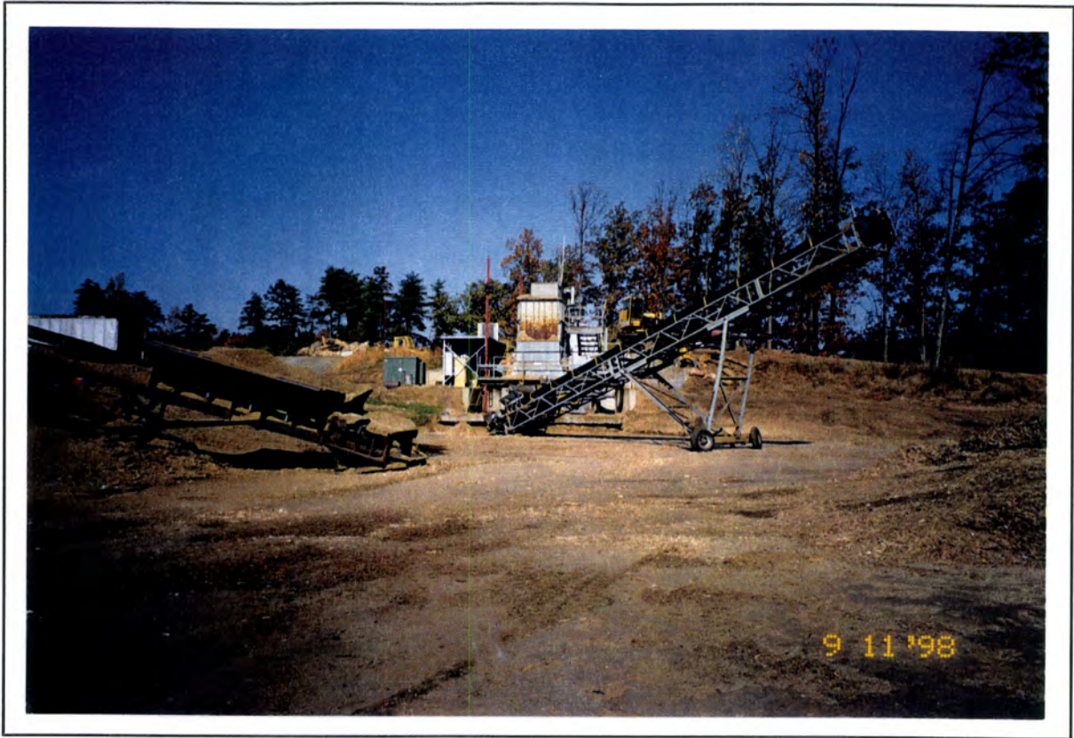
Radial Stacker from Processing Unit to Stock Piles, looking north.
